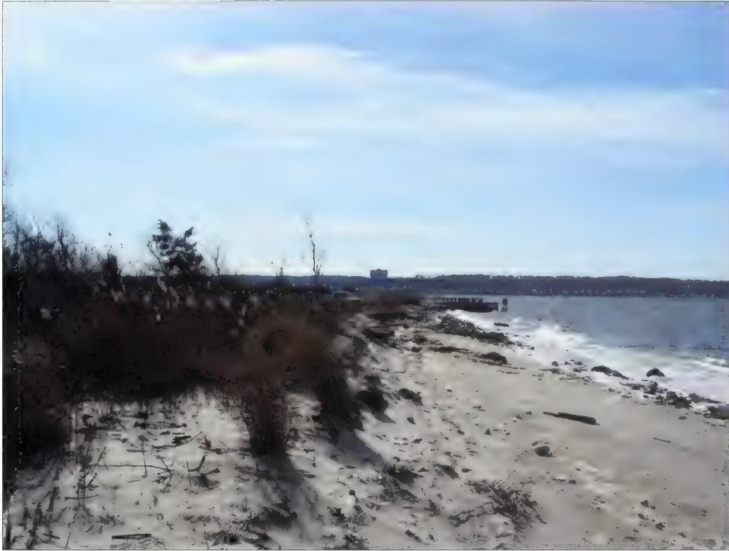
Figure 3.45. View looking south at eroded vehicular route, Battery Mills. On the west side of Battery Mills a portion of the road encircling the battery, approximately 200-feet, has been washed away by Sandy Hook Bay (Olmsted Center, January 2009).
